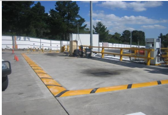
The AWIS Preform highlights the bunded area and as it is anti slip it is safe to walk over and the retroreflectivity allows it to be identified when the headlights of the buses shine on it.
