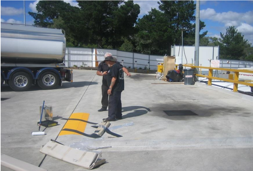
The refueling bunded area. It is very hard to identify the raised bunds.
