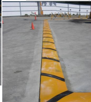
The AWIS Preform highlights the bunded area and as it is anti slip it is safe to walk over and the retroreflectivity allows it to be identified when the headlights of the buses shine on it.
