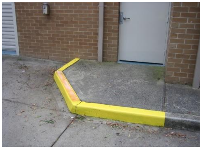
AWIS Preform Treatment of kerbs
