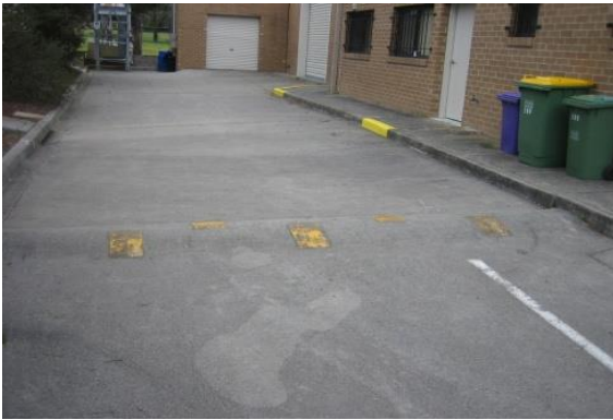
A speed hump the paint has degraded new Anti Skid AWIS Preform installed
