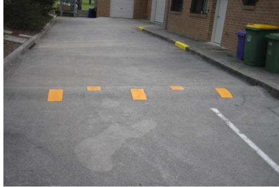
A speed hump the paint has degraded new Anti Skid AWIS Preform installed
